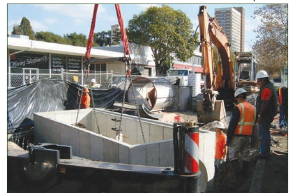
Installation of a trash separator
