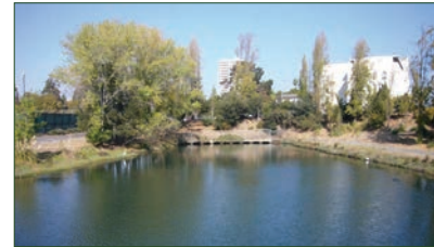
Existing 10th street culverts
